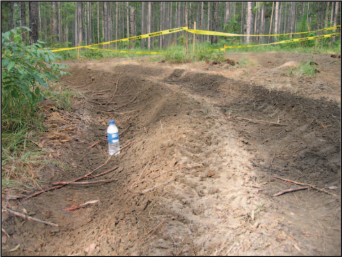
Figure 54—Loop B, 8-inch rut on the turn.
