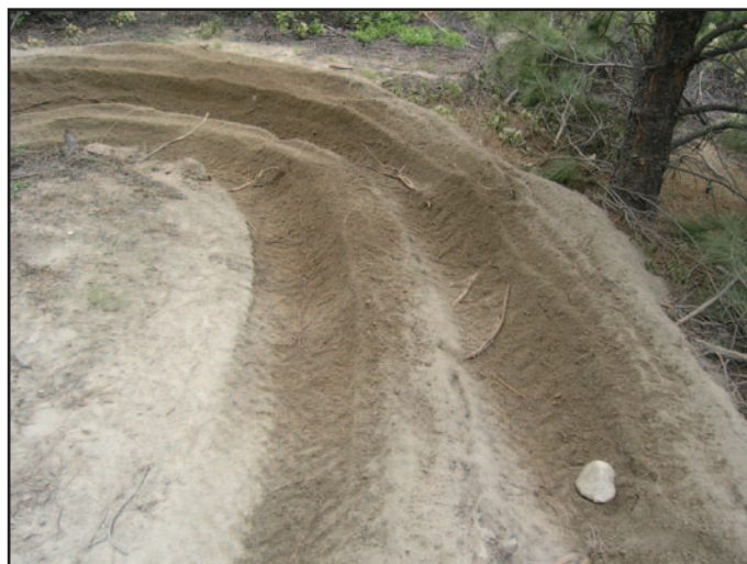
Figure 90—Loop D turn, rut depth 10 inches.
